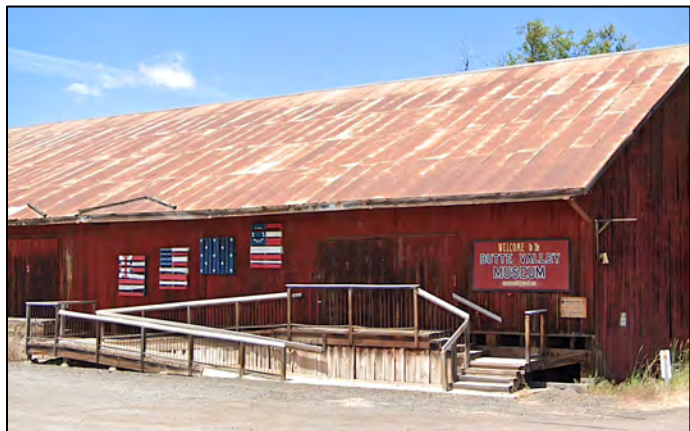
Figure 5-4, Butte Valley Museum at the former mill site
